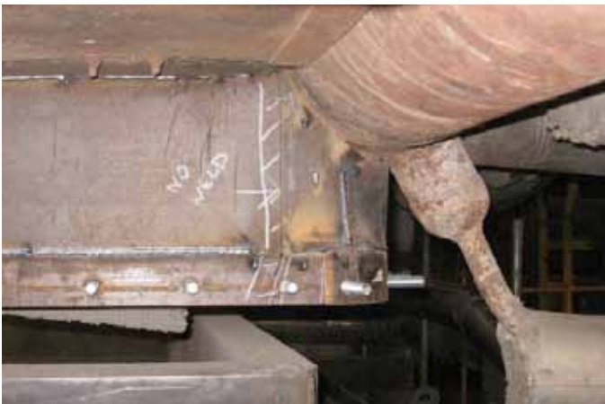
Installation of DEKOMTE steel parts
