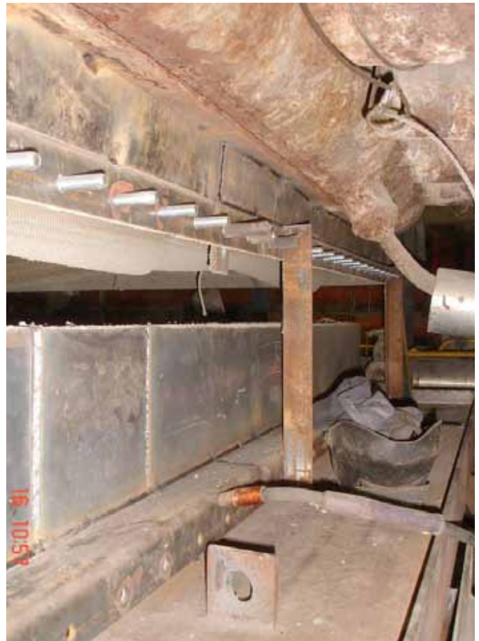
Installation of DEKOMTE fabric joint
