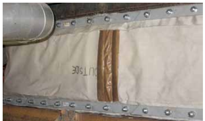
Installation of DEKOMTE fabric joint
